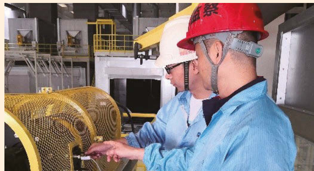
• Screening and handling of hidden safety hazards and the corresponding subsequent review on such work
